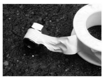
USING AN ADJUSTABLE SPANNER WIND THE HEX BUSH CLOCKWISE INTO THE VALVE ASSEMBLY. WHETHER IT TIGHTENS AT A POINT SOME OR ALL OF THE WAY IN DEPENDS ON THE COMBINATION OF TAPER OR PARALLEL THREADS. IF THE HEX BUSH DOESN'T FIT THEN SEE THE TROUBLESHOOTING SECTION AND APPENDICES FOR ALTERNATIVES. THE CONNECTING THREAD WILL ALMOST ALWAYS BE A 1/4" BSP.
